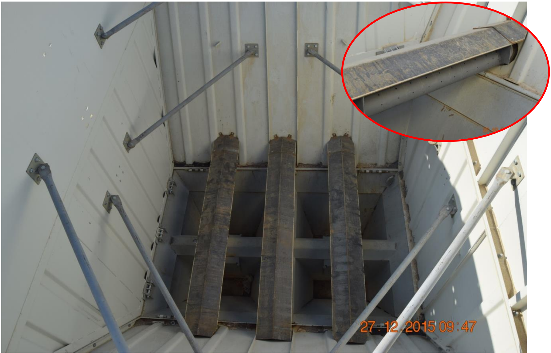
Air pipes inside the coarse aggregate bins
