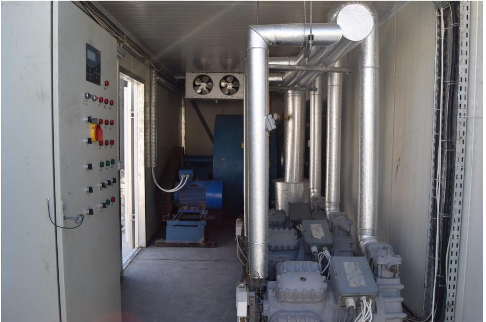
Refrigerating system and control panel-Automated system
